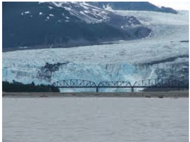
Figure 3 Million Dollar Bridge with Glaciers Behind (3 of 4 spans).
