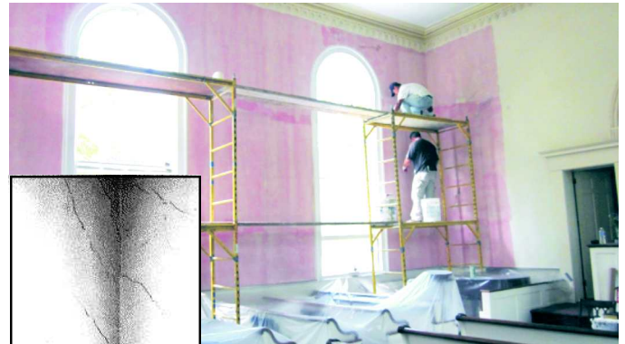
Plasterer repaired cracks and applied special finish to minimize future cracking and crazing.
