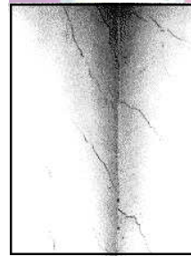
Plasterer repaired cracks and applied special finish to minimize future cracking and crazing.
